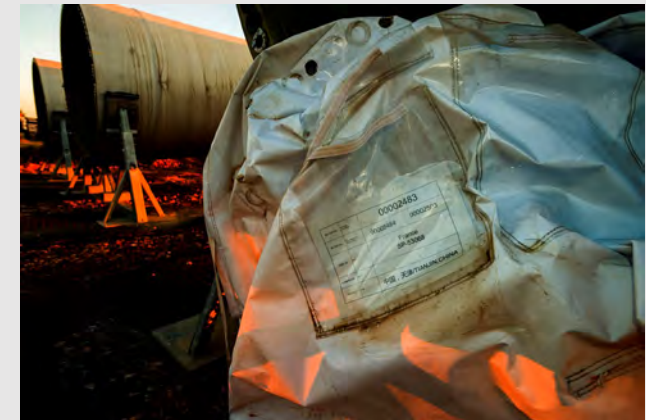
Tarps covering the blades of the Sainte-Victoire wind turbines bearing the words “TIANJIN CHINA”
